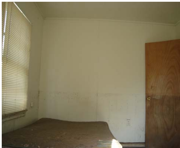
Figure 2-3: Interior Mud Line HWM
